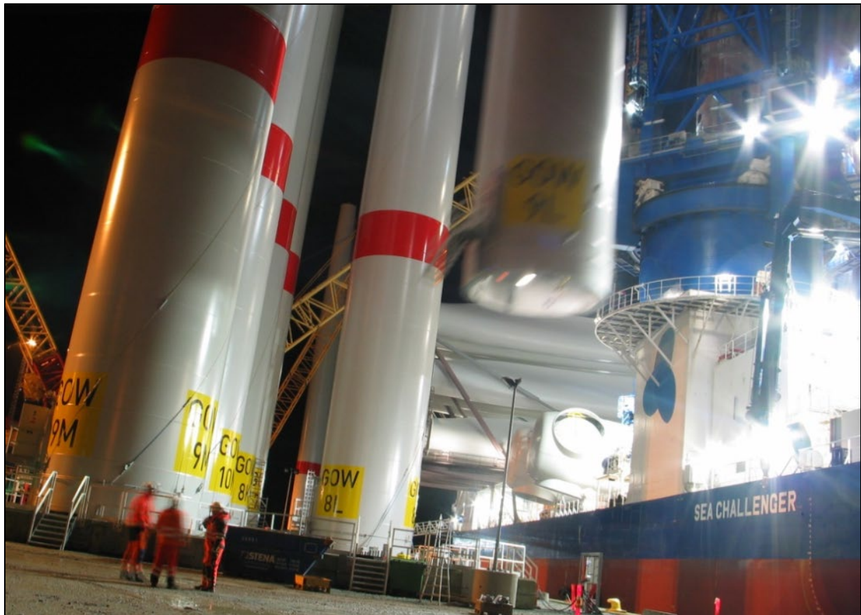
Figure 10.9 Loading Towers onto Installation Vessel (Gode Wind, 2015)
